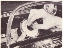
Connect the battery cable. With the ignition turned "ON", turn the tester pointer first to "L", next to "M" and then to "H". The gauge should read, in succession, at the low end, the middle, and then the high end of the scale.
